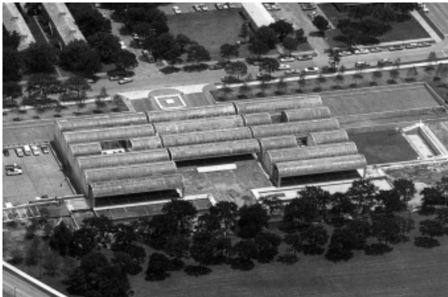
Figure 1.2: Aerial photo from the west during construction, June 1972 [Fra99]
